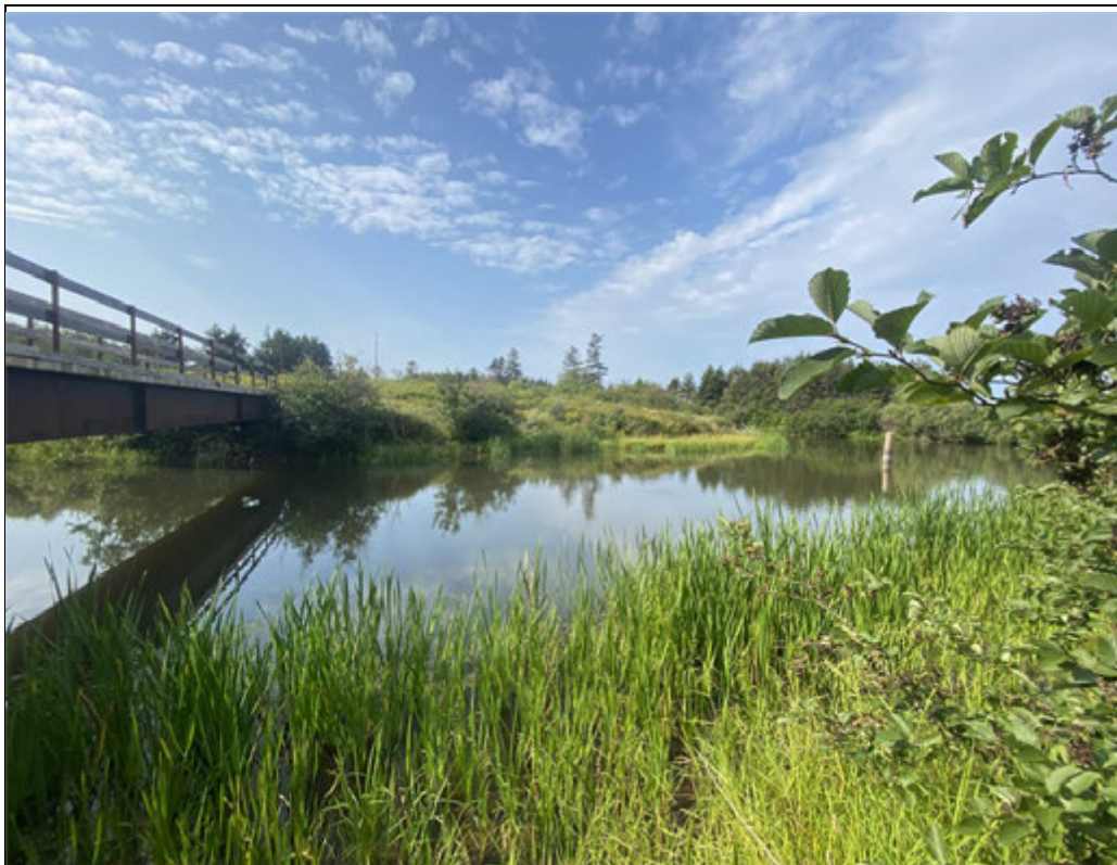
Photo 20: MT-2 26 Aug 2021 Direction: Southwest
